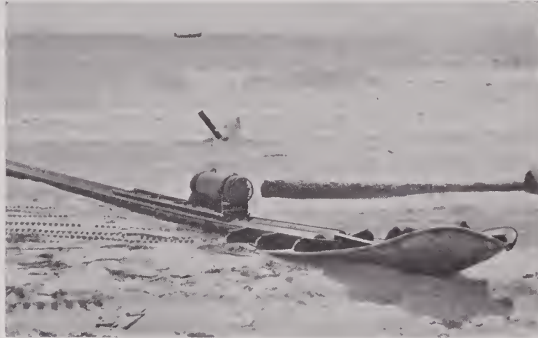
FIGURE 13. Snake with special bow attachment on beach at Fort Pierce, Florida, after offshore launching.
